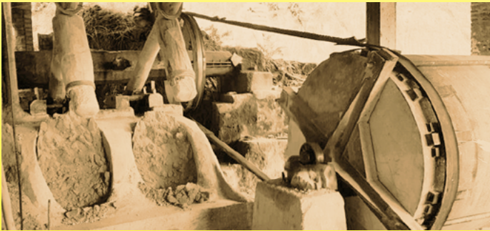
Traditional production machines ((水碓 shui dui) for production of powders used to make electric porcelain (private collection)
