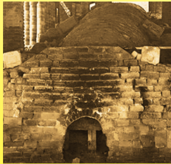
Traditional Chinese Dragon oven (龙窑 Long Yao), feeding mouth and filling method with electric porcelains (private collection)
